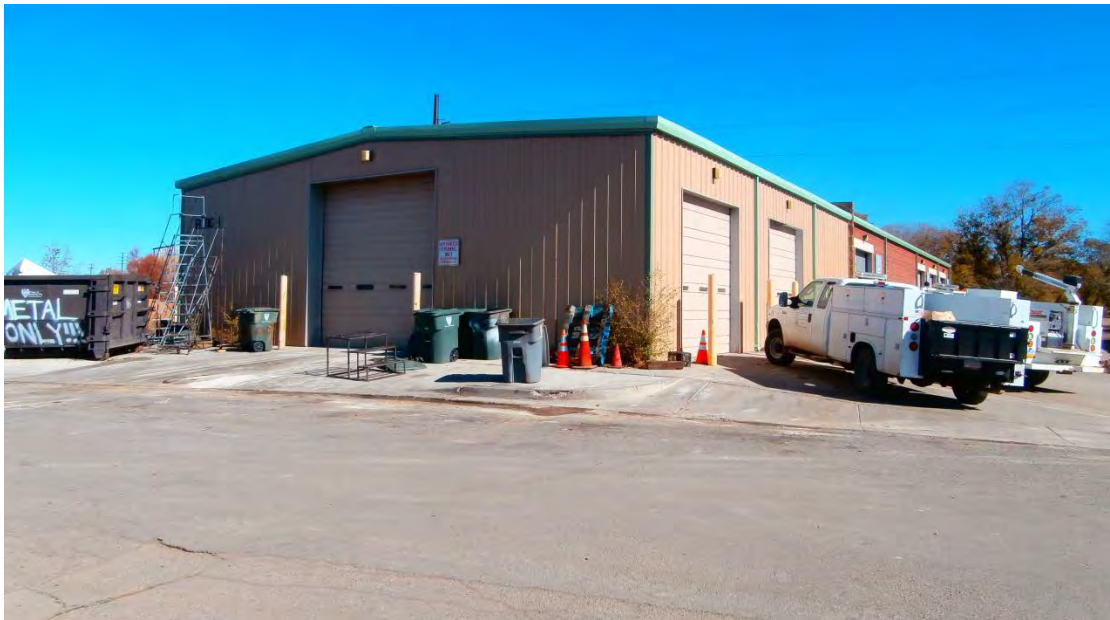
Figure 4-1. One Bay Fleet Maintenance Shop Exterior
