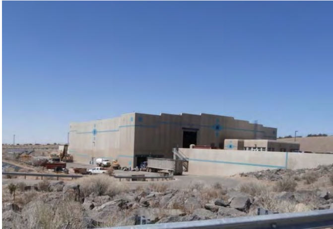
Figure 3-8. Transfer Station (Note Tractor-Trailer Entering Lower-Level Tunnel)
