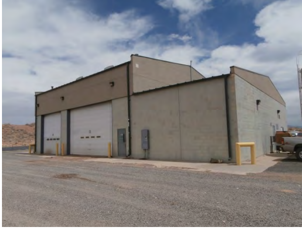
Figure 2-2. Fleet Maintenance Building
