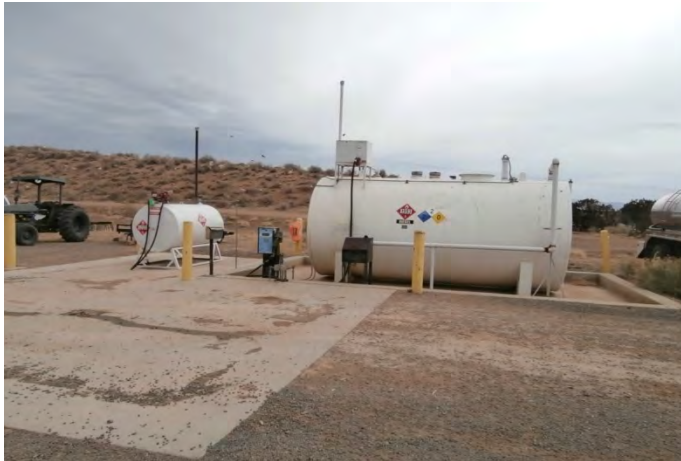
Figure 2-3. On-Site Fuel Storage
