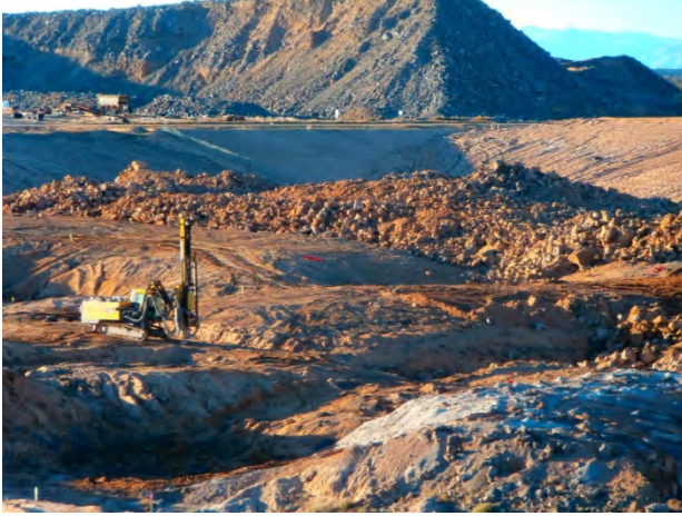
Figure 2-8. Drill Rig Preparing Bore Hole for Blasting in Front of Blasted Rock
