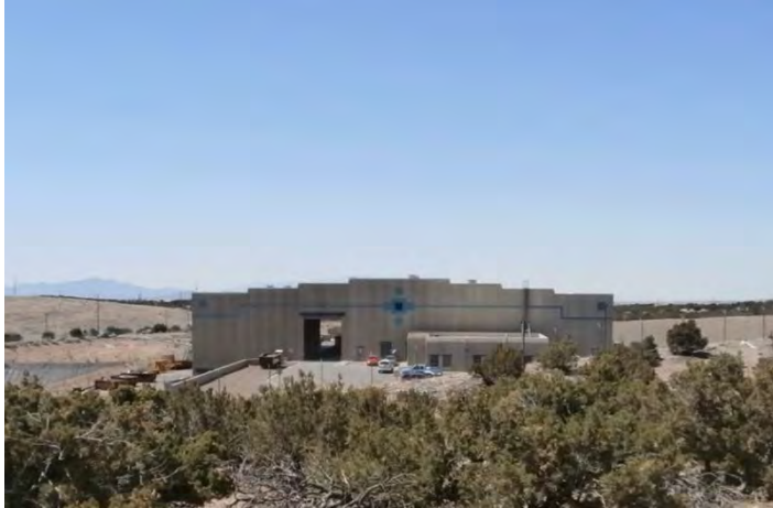
Figure 3-5. Transfer Station Building
