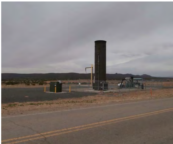
Figure 2-7. Landfill Gas Flare
