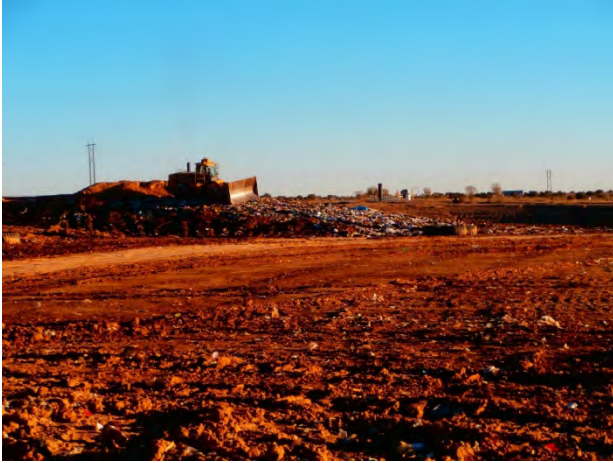
Figure 2-4. Landfill Compactor Operating on Work Face
